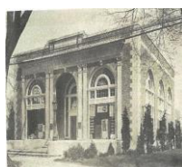
Clinton Light and Power Company
